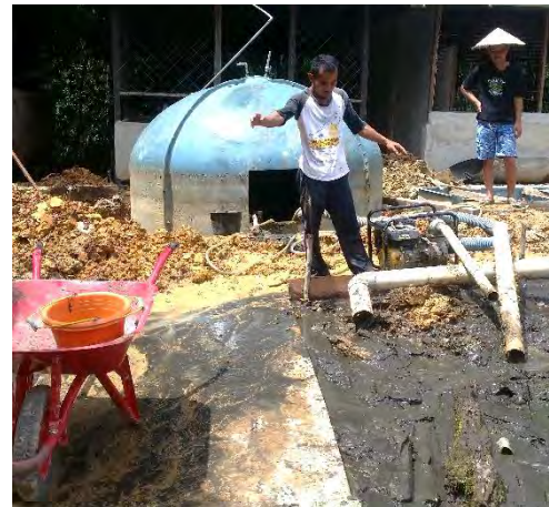
Installation of biogas production system at Sadap village
