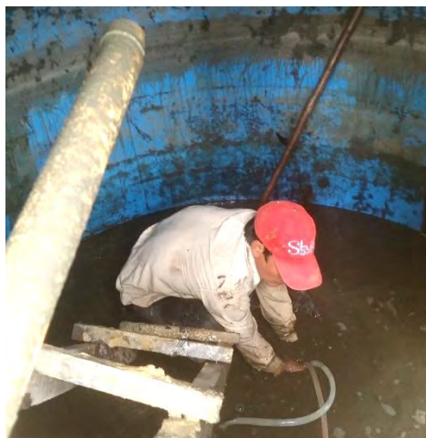
Installation of biogas production system at Sadap village
