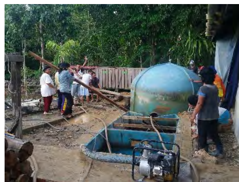
Installation of biogas production system at Sadap village
